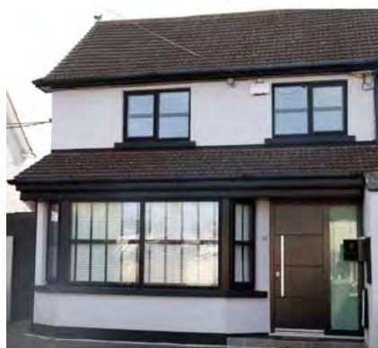
Front of house, after renovations
